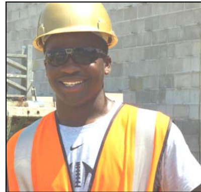
2011 graduate Timothy Jones interns for the City of St. Louis Civil Engineering Department at the O'Fallon Recreation Center project site.
